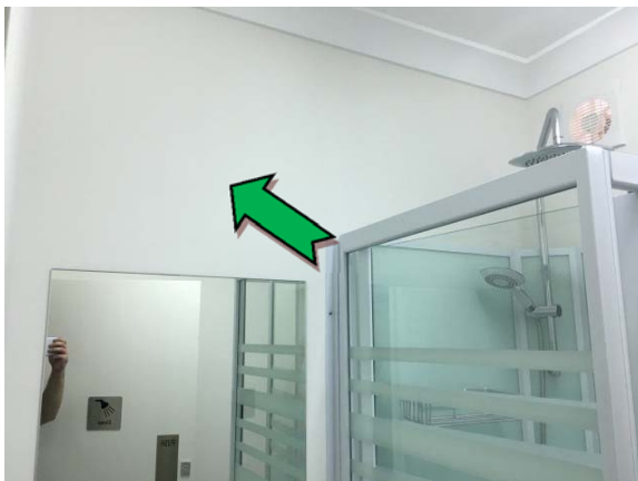
Photo 5. Interior, shower room, north elevation, wall – non asbestos-containing fibre cement sheeting.
