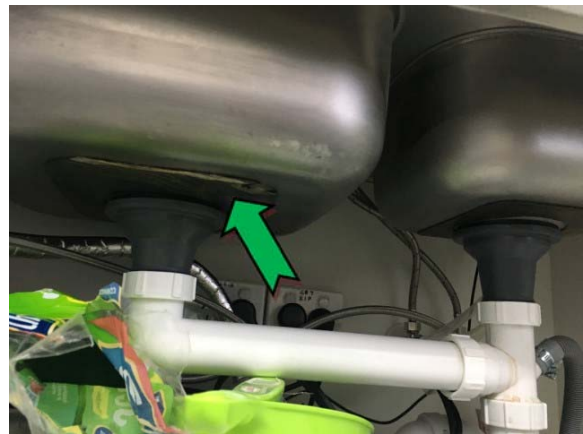
Photo 4. Interior, kitchen, sink pad – non asbestos-containing bituminous material.
